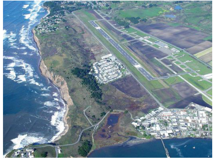
Half Moon Bay Airport aerial view.
